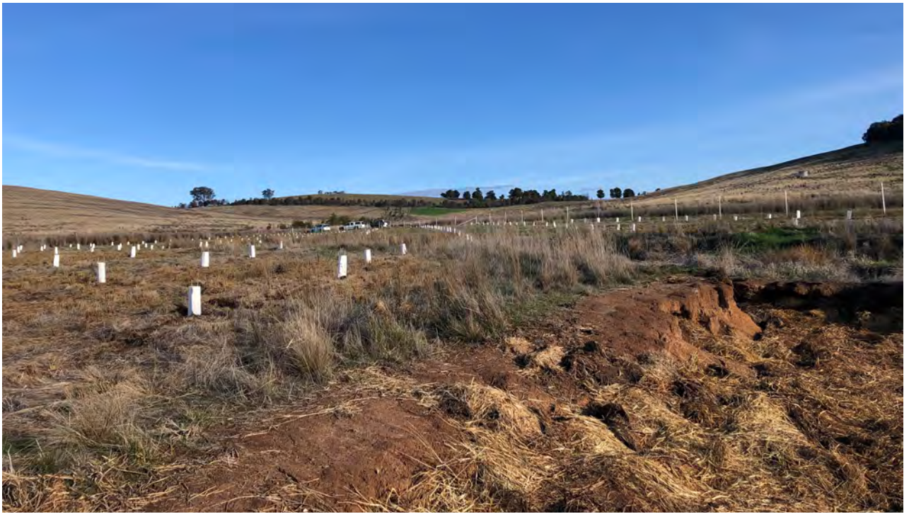
Figure 14: Erosion revegetation using mulch. Photo: Kathie Le Busque
