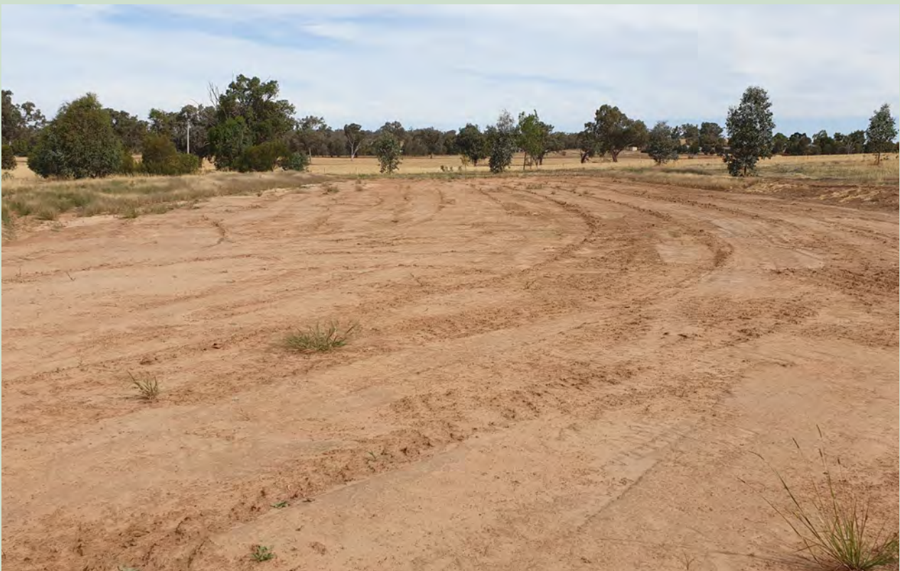
Figure 31: Scalping of a site for groundlayer restoration with the top 10–15cm of soil removed from a highly degraded site. Photo: Sue Rose
