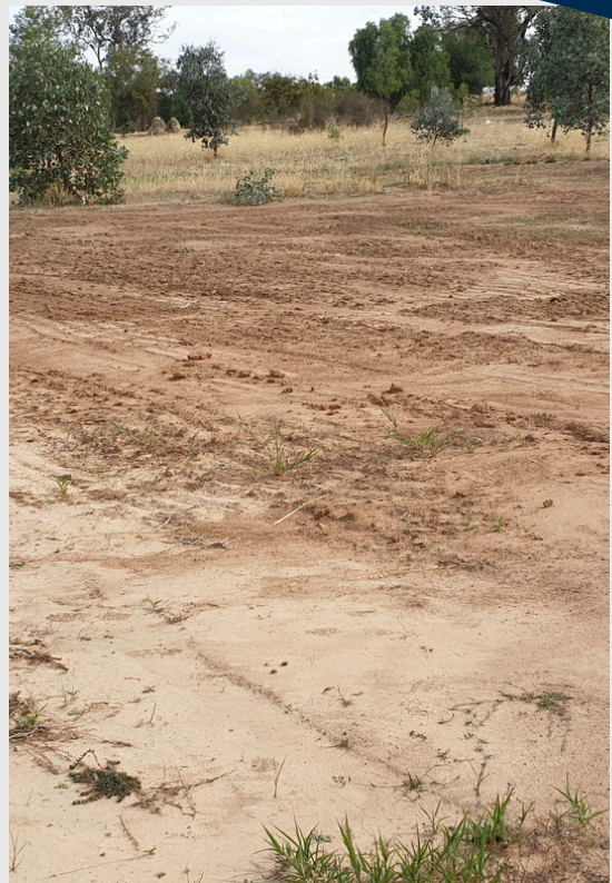
Scalped topsoil 10-15cm
